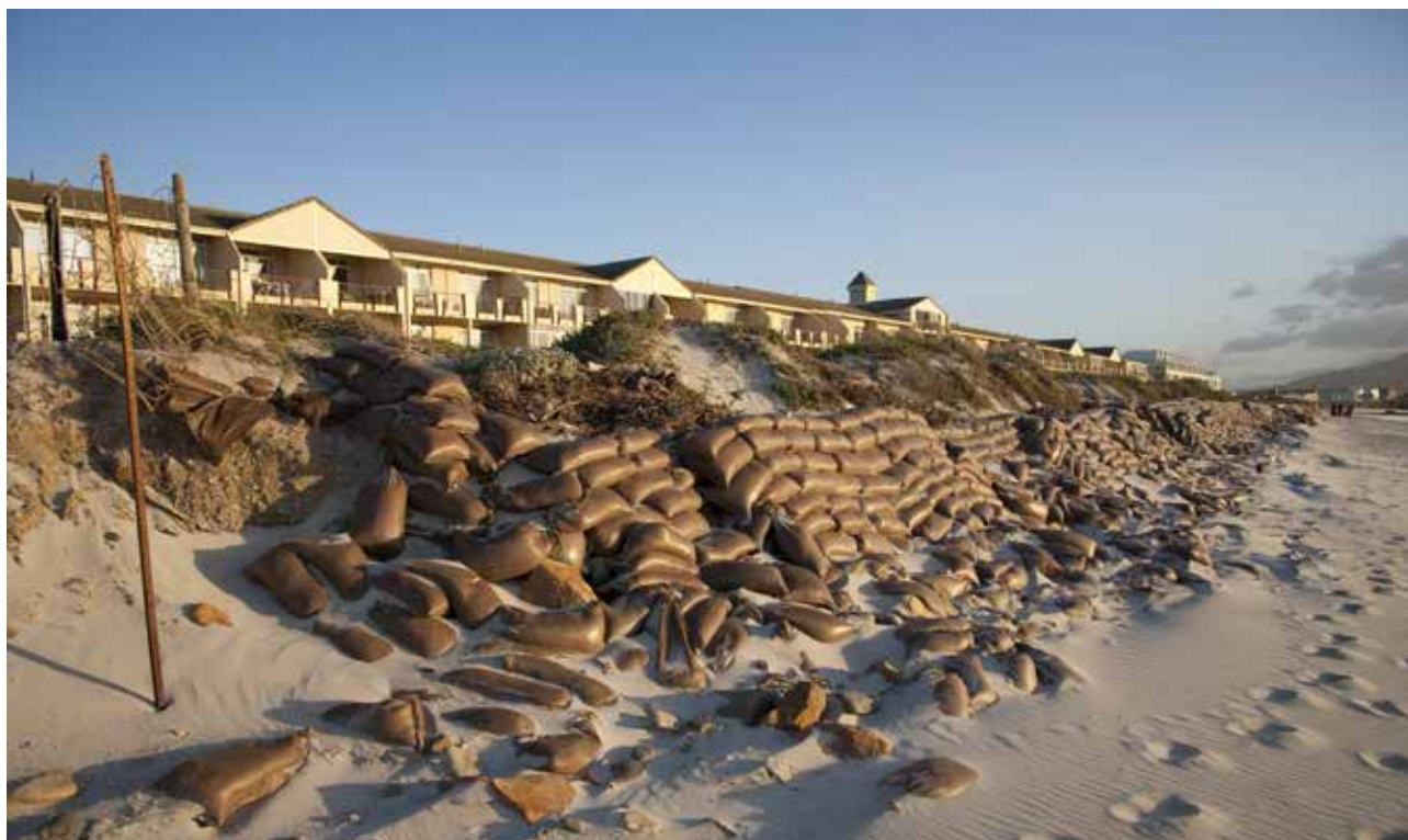
Coastal erosion and inefficient erosion reduction measures at Cape Town, South Africa. © 2009 SEI/Sean Wilson
