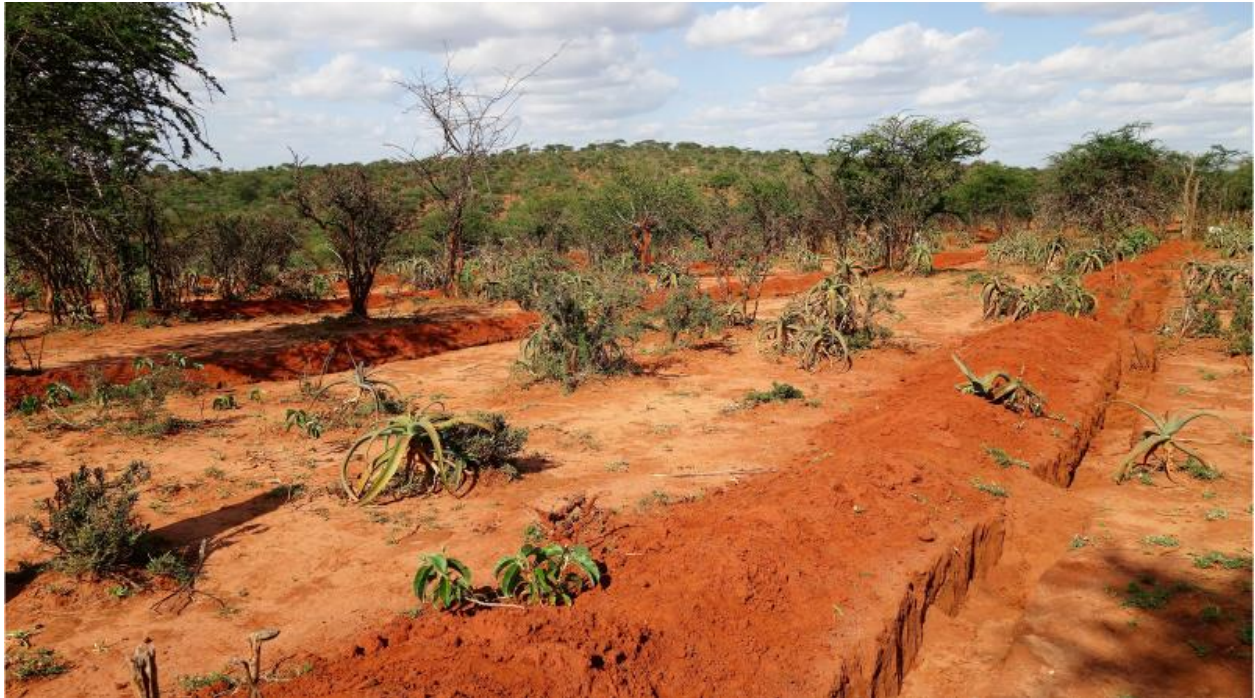
Photo Note 4. Soil bunds (trenches) to capture rainfall on parched land in Nanawa grazing area in Yabelo woreda. The soil bunds were dug by hand in a collaborative effort among different ethnic communities. Photo by Katsuaki Terasawa.
