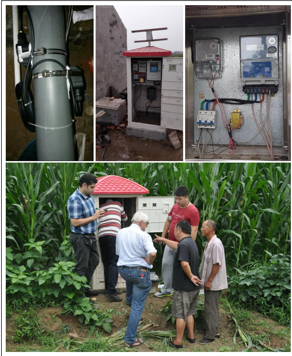
Figure 49: Hengyuan meter and RSA meter. Upper left: The Hengyuan ultrasonic water meter; Upper middle: The meter is protected by a cement box. The control box and data transmission unit is protected by a plastic hut; Upper right: RSA meter box; Bottom: Swiss expert answered questions from the local farmers during the installation of RSA meters by technicians from RSA and local DWR.
