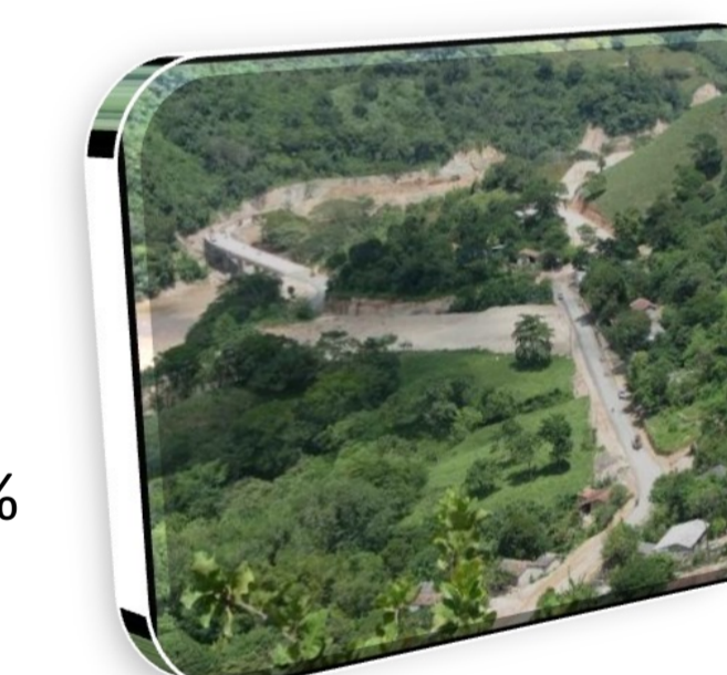
New Northern Highway, 184 kms of deforestation in the area with higher national levels of annual precipitation
