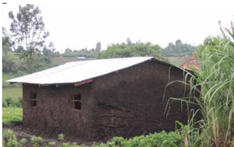
Picture 3. Manure used as construction material
