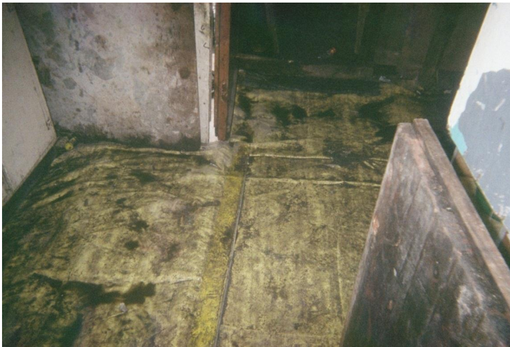
Picture 10: Putting plastic on floor: “At the back, water coming through the floor, here they have put plastic on the floor to keep it out.” (Flooding observer 19.6.2011)
