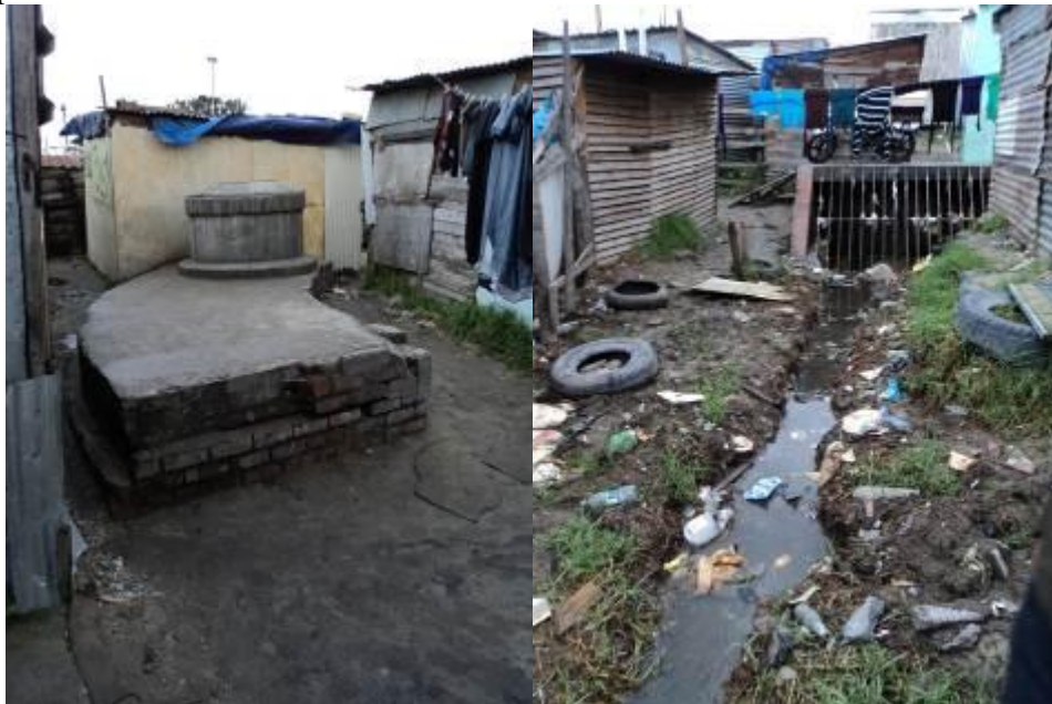
Picture 2: Open sewer manhole in the middle of the settlement, which overflowed during the winter of 2009 Picture 3: Storm water / sewage pipe with a grating. People throw waste and buckets with toilet sewage into here (since there are so few toilets in the area, many use buckets). I have not observed similar structures in any other settlements. 22.08.2011.
