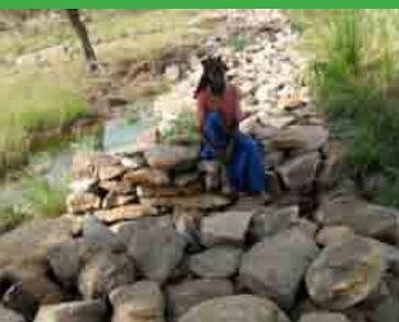
Fig.4. Dike for water retention in Mali
