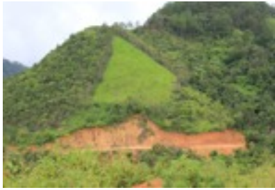
Evidence of Landslides, Kon Tum Project Site
