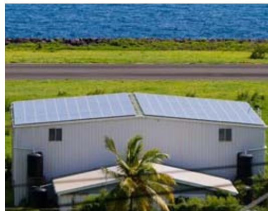
Figure 2: Hangar at Bequia Airport with solar panels installed on the roof
