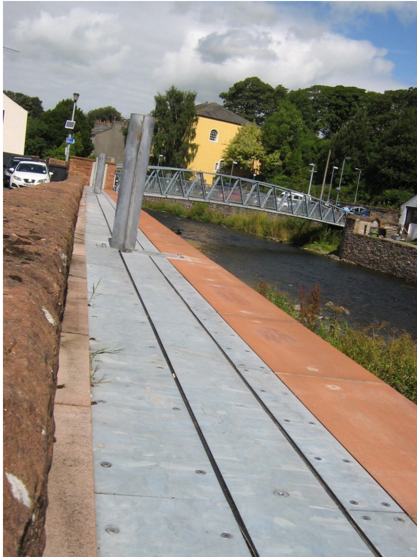
Plate 6.6: Cockermouth automatic flood barrier © H Deeming 2014
