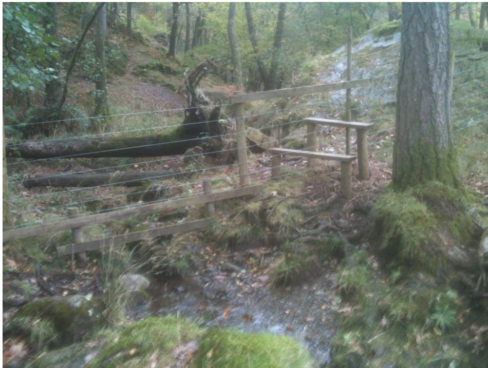
Plate 6.1: 'Flood resilient' Single strand fencing (Borrowdale) ©H Deeming 2014
