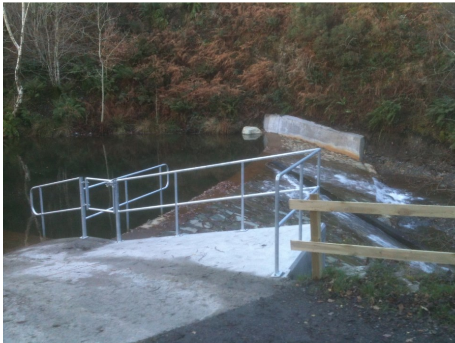
Plate 6.2: Braithwaite Sediment Catch Pit (note fish ladder) ©H Deeming 2013
