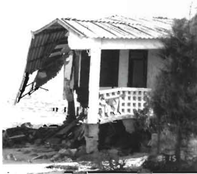
Fig. 4. Houses are damaged due to continued beach erosion in Unit 3, Banjul to Cape Point
