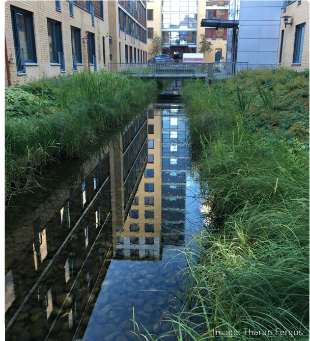
Open retention basin for stormwater in the student city of Bjølsen
