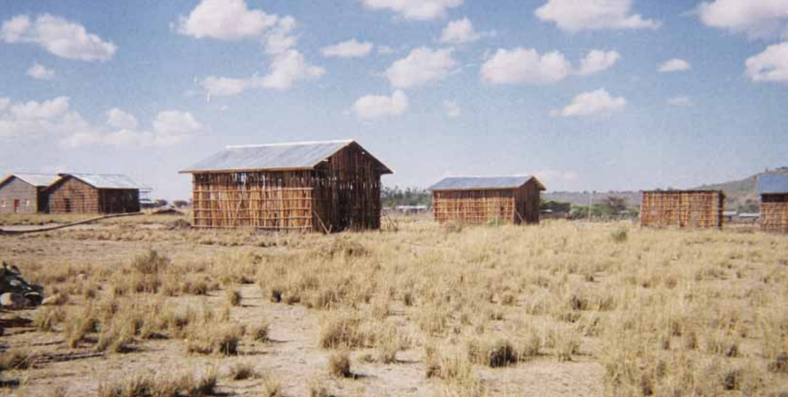
Rural SNNPR housing construction, Sidama Zone, Loko Abaya Wereda.
