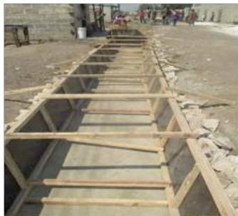
Concrete lining of the drainage.
