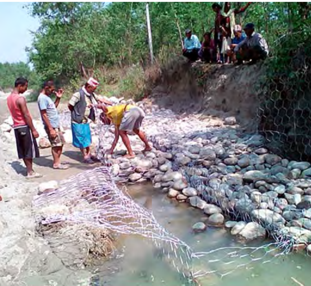
NEPAL: Riverbank stabilization project in Nepal to address increased erosion. One aspect of this project is that it uses locally-available materials. Another is that the project improvements can be maintained locally.
