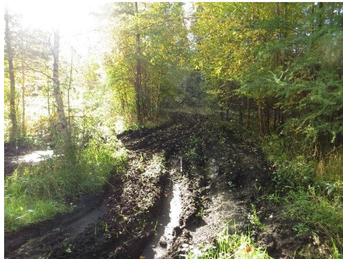
Figure 14. Example of soil rutting and compaction
