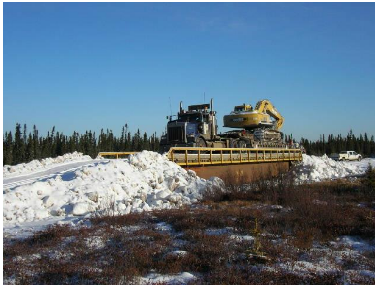
Figure 25. Bridge in place (photo credit Millar Western)
