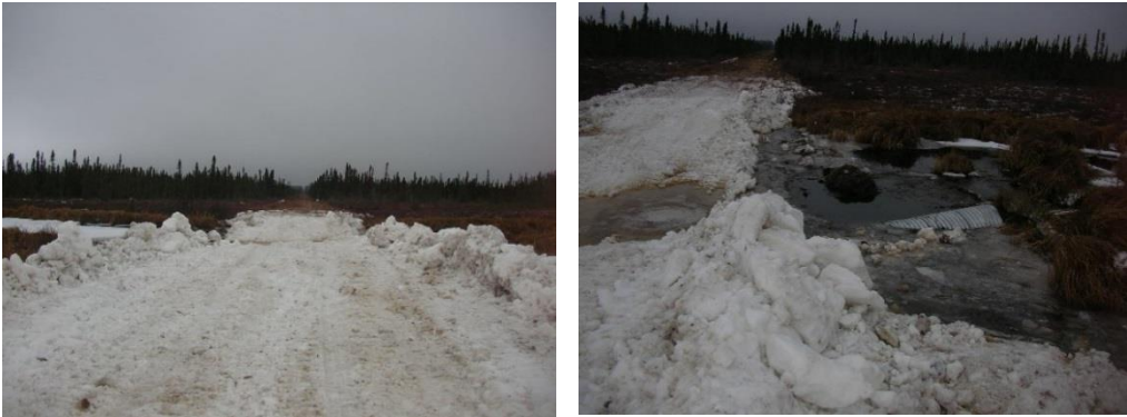
Figures 21 and 22. Snow bridge and culvert (photo credit Millar Western)
