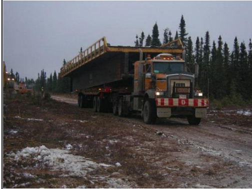
Figures 23 and 24. transporting and placing the bridge (photo credit Millar Western)
