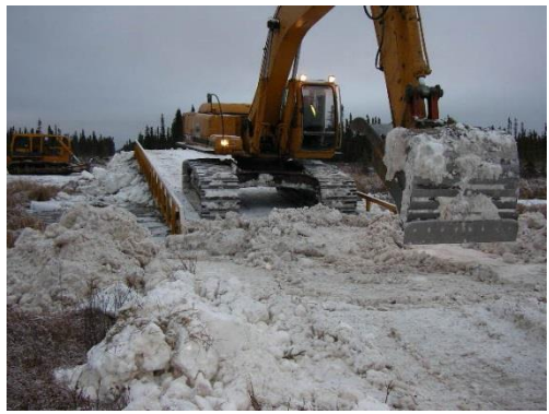
Figures 23 and 24. transporting and placing the bridge (photo credit Millar Western)
