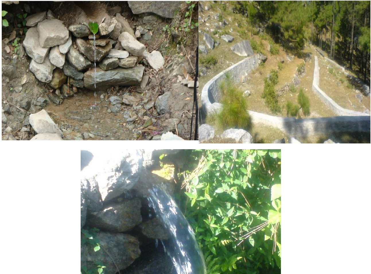
Figure 9: Photographs of Spring Rejuvenation done by BARC in Uttarakhand a. Drying Spring b. Water recharge through constructing water harvesting structures c. Rejuvenated Spring
