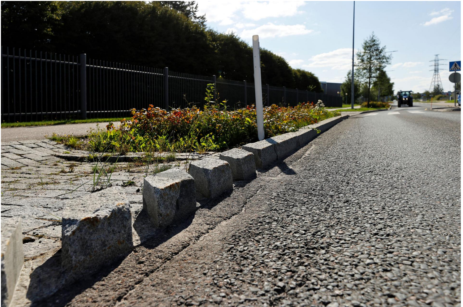
Figure 34. Different types of kerb were tested in the Meiramitie road biofiltration swales to determine which solution directs the stormwater more effectively. This swale has openings in the curb. Photo: Mikko Käkälä /HSY.
