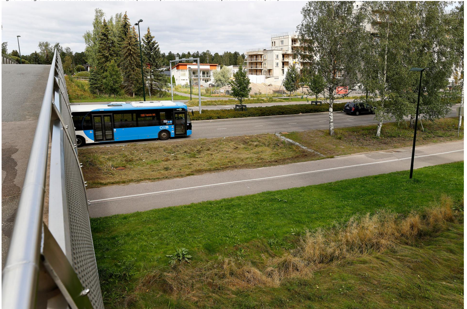
Figure 26. The vegetation in the biofiltration area on the south side of Merituulentie road has not thrived and new plantings were foreseen in the autumn 2021. Photo: Mikko Käkela/ HSY.
