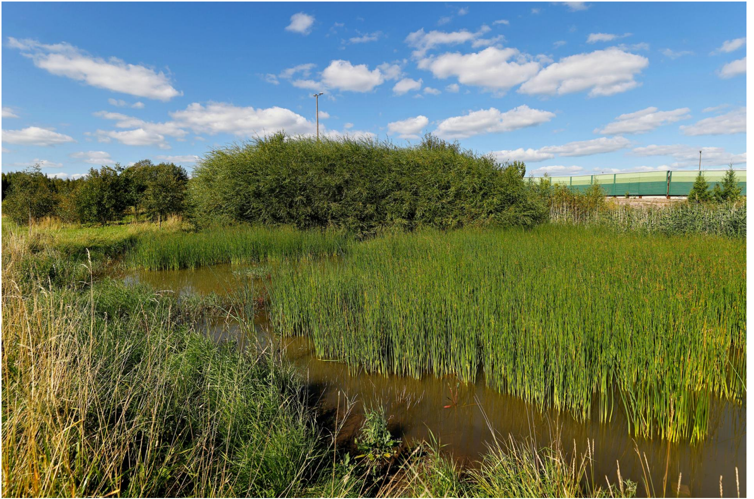
Figure 29. The biofiltration area purifies the snow melt water of the Koisoitie road snow reception area of which green rampart can be seen in the background. Plants include common reed, common club-rush and narrowleaf cattail. Photo: Mikko Käkälä/ HSY.
