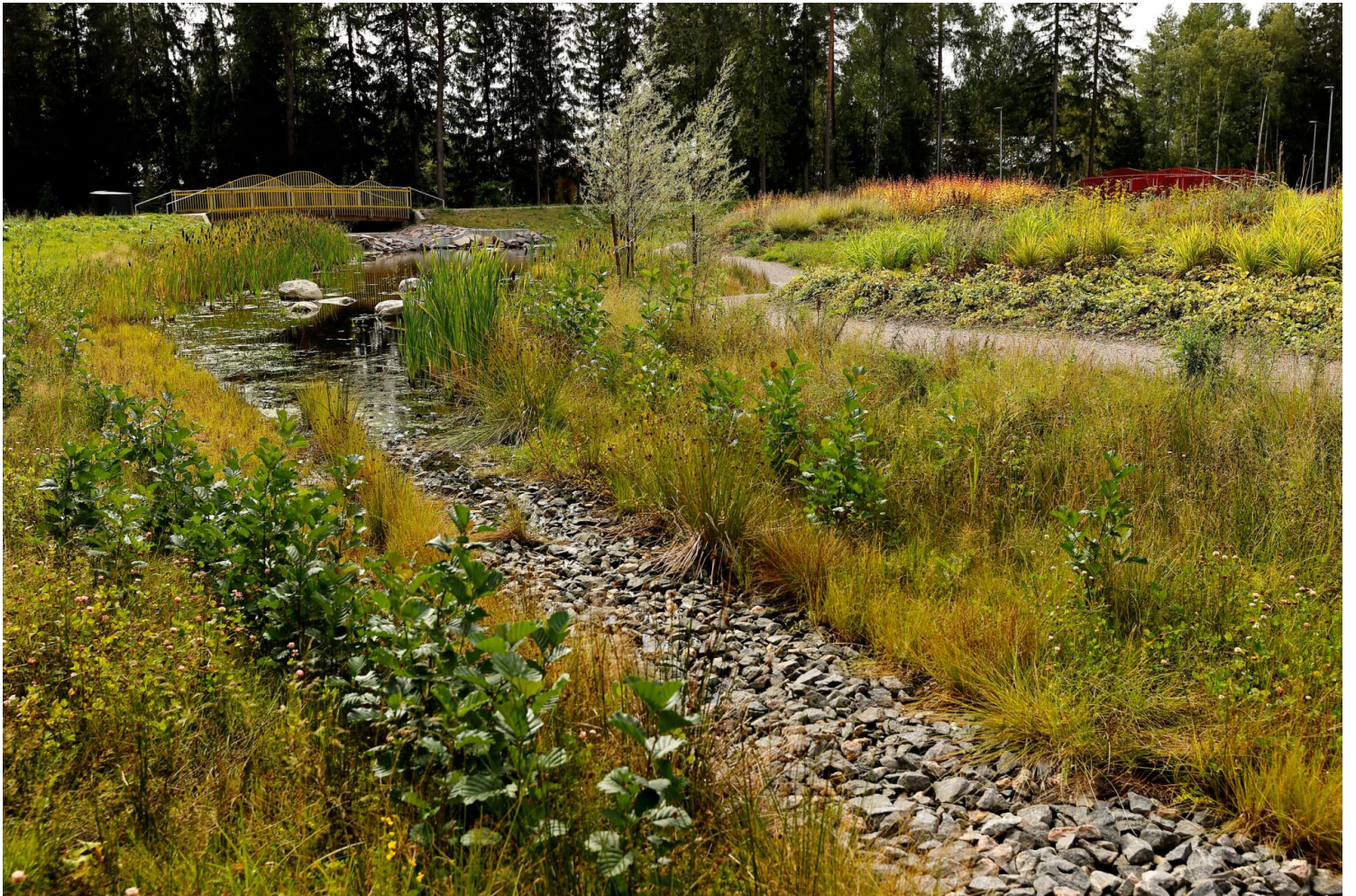
Figure 14. Water is conveyed to the wetlands through meandering channels that are partly wetland-like or grass covered depressions, partly streams with gravel or rock surfaces. Photo: Mikko Käkälä /HSY.
