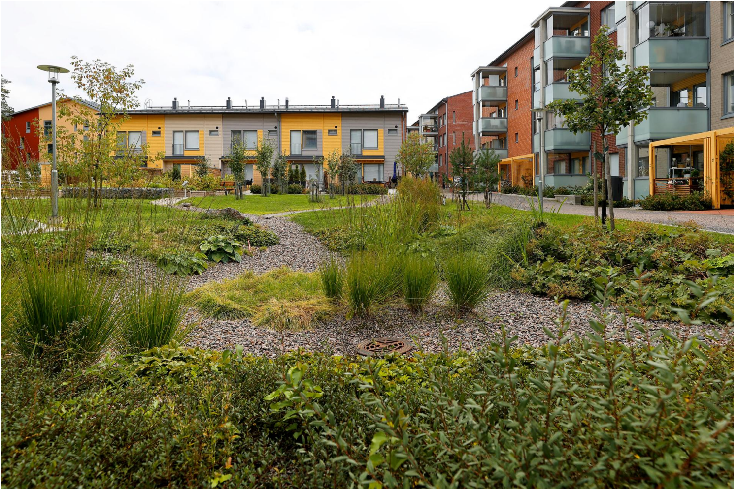
Figure 11. In the Fannynkallio residential area the topography was designed so that surface waters are directed to the rain gardens. Photo: Mikko Käkälä /HSY.
