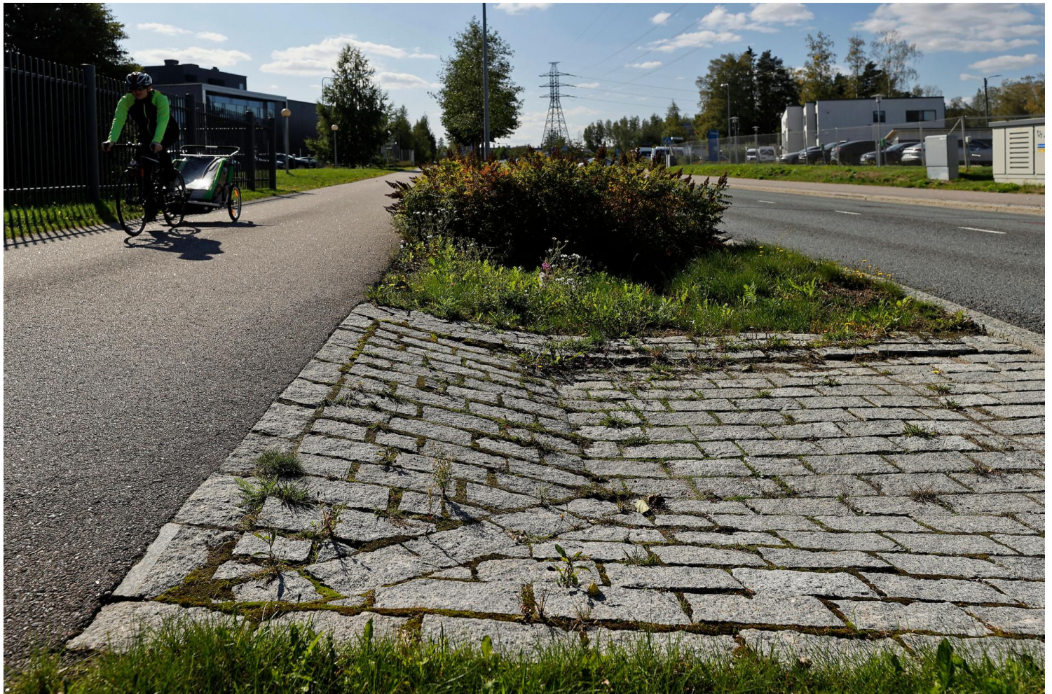
Figure 33. Stormwaters are directed with road levelling onto the paved depressions retaining the water, which collect the suspended solids and rubbish conveyed with the stormwater. Photo: Mikko Käkälä /HSY.
