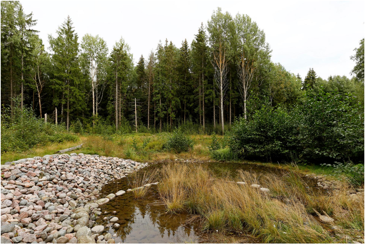
Figure 16. The stormwater management system of Maunulanpuisto park consists of a sedimentation basin and a biofiltration area. Photo: Mikko Käkälä /HSY.
