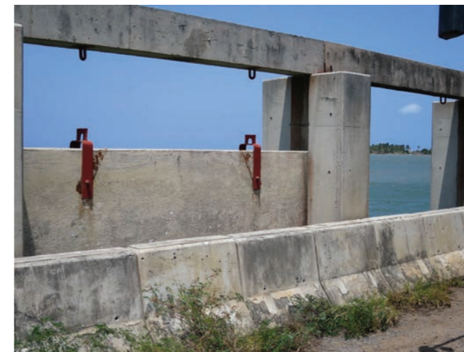
Volta sluice gate (Photo: Katharine Vincent)
