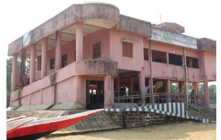
Cyclone shelter in the Mahanadi (Photo: DECCMA India)
