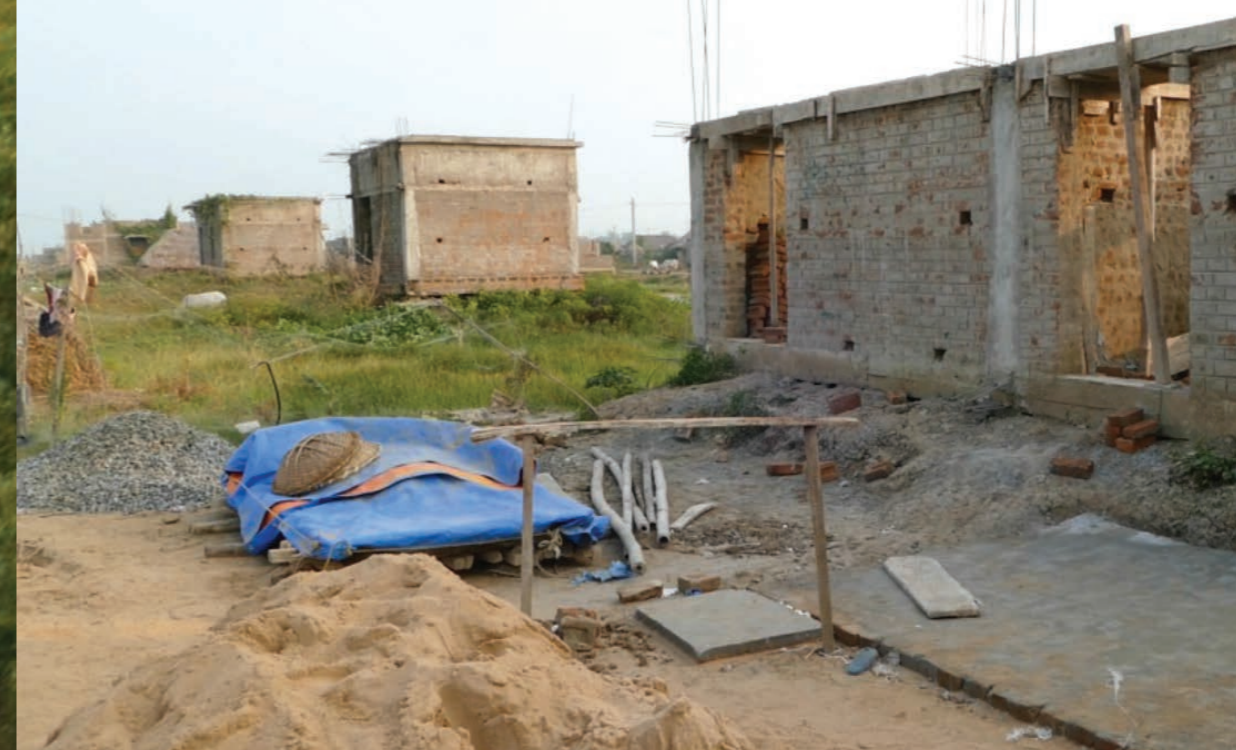
Houses under construction in Bagapatia.
