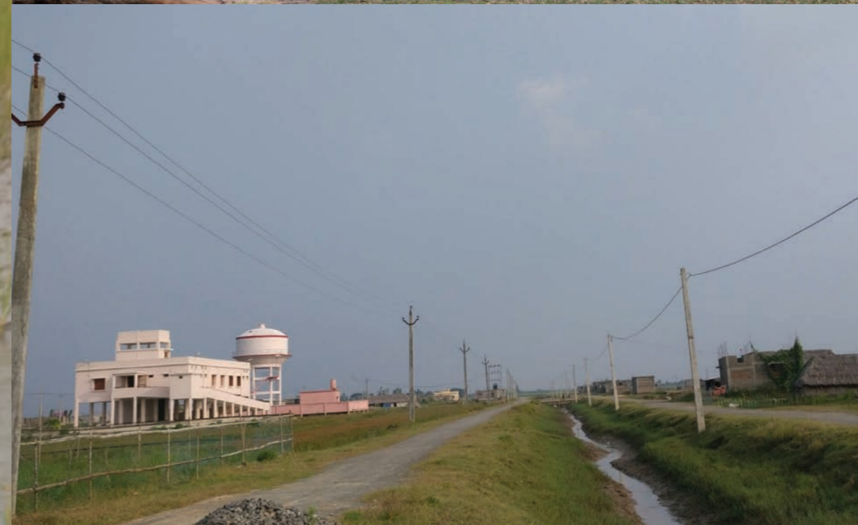
Overhead tank for drinking water, cyclone shelter, and electrical lines at Bagapatia
