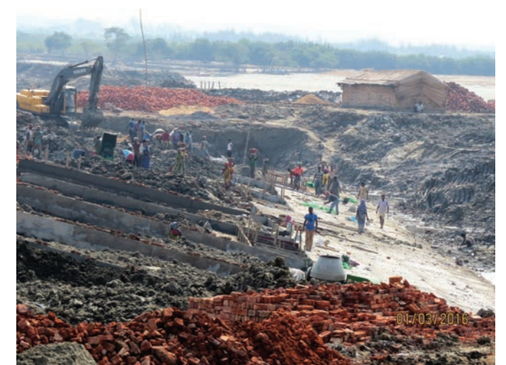
Embankment construction in the Indian Bengal delta (Photo: Shouvik Das)
