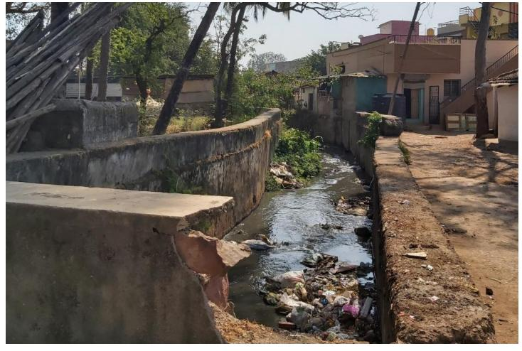
Concretised drains clogged with solid waste exacerbates flooding incidents inside the settlement. Haveripete, Dharwad.
