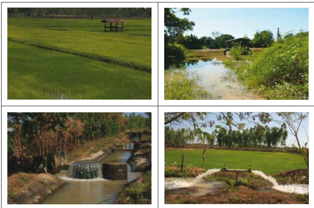
Figure 5: Dry-season rice farming is the development plan's key strategy. The irrigation system pumps from the river (the top right image shows a pump station) through underground pipes to the rice paddy (bottom left & right).
