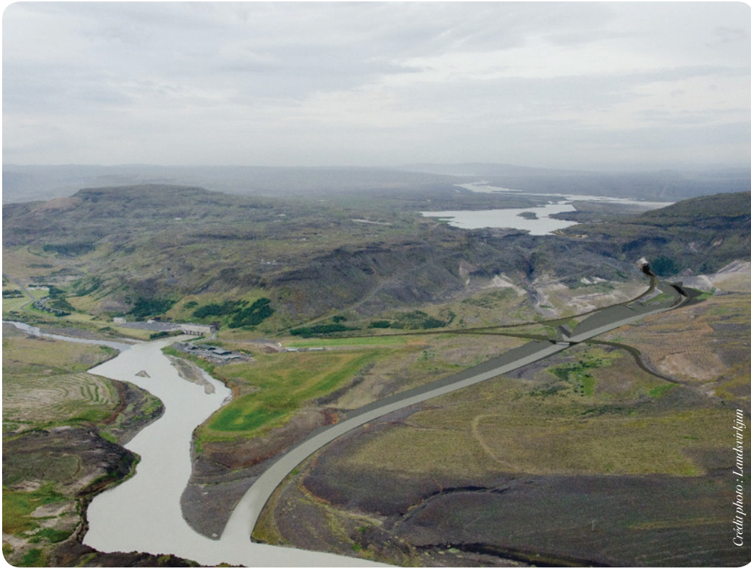
Figure CS2.4 Graphic modelling of the projected underground expansion of 100 MW at Búrfell generating station. The left side of the picture shows the old Búrfell generating station and the right side shows a computer drawing of the projected discharge channel of the underground generating station.
