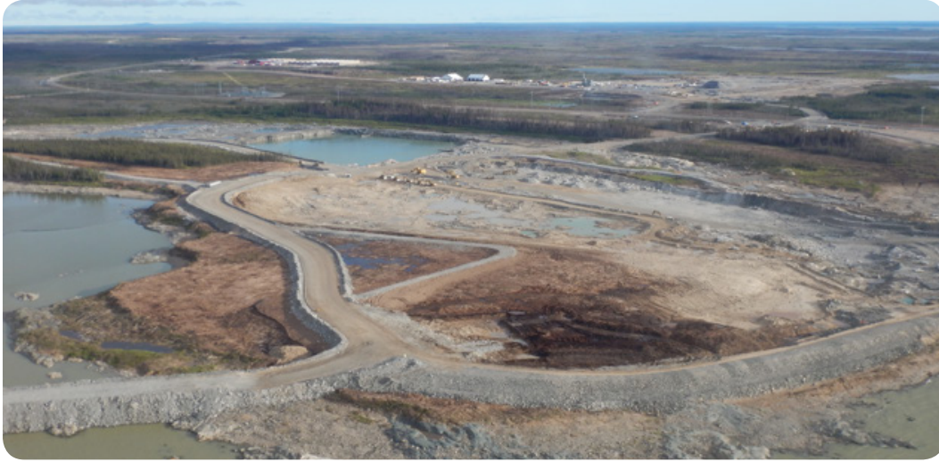
Figure CS4.5 Keeyask Construction Site Photo (June 21, 2015)
