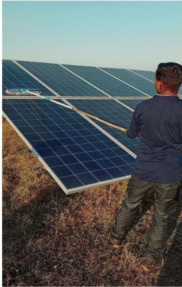
FIGURE 19. Solar panels being cleaned.
