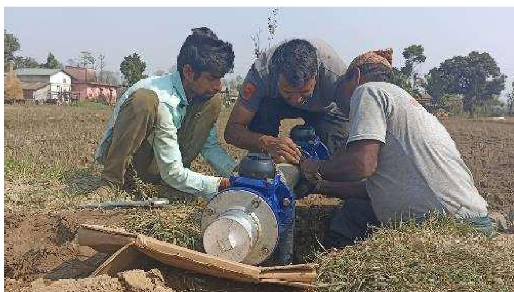
Fixing of meter in the pump
