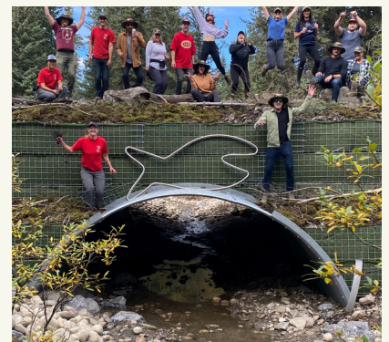
Culvert replacement Trout Unlimited Canada
