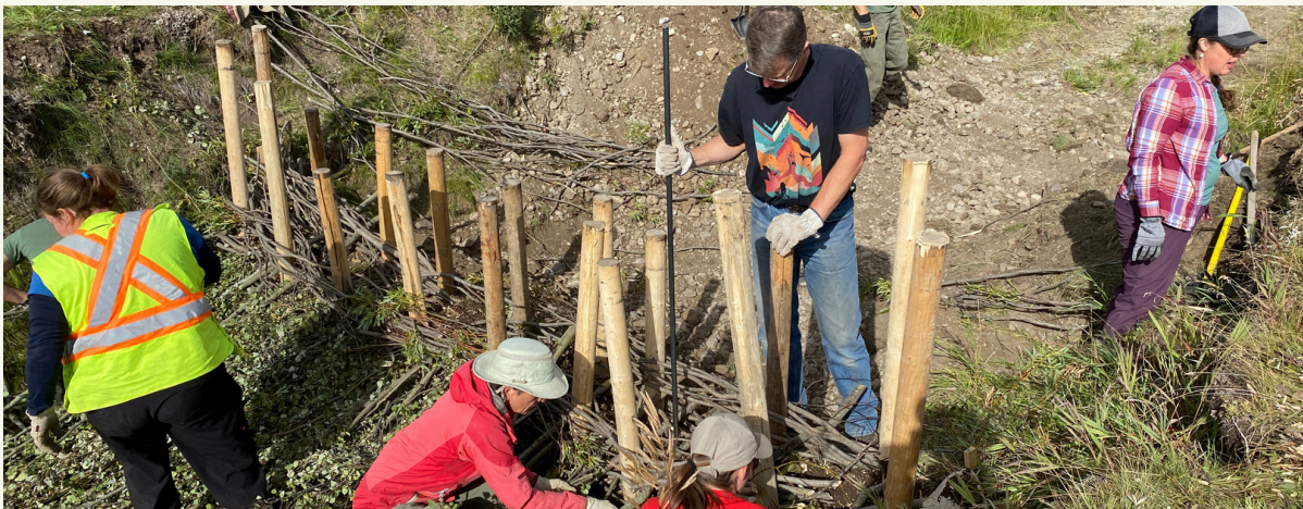
Constructing a beaver dam analogue. Courtesy of Trout Unlimited Canada
