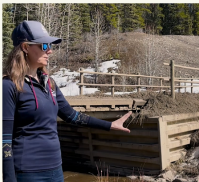
Bridge re-construction Elbow River Watershed Partnership
