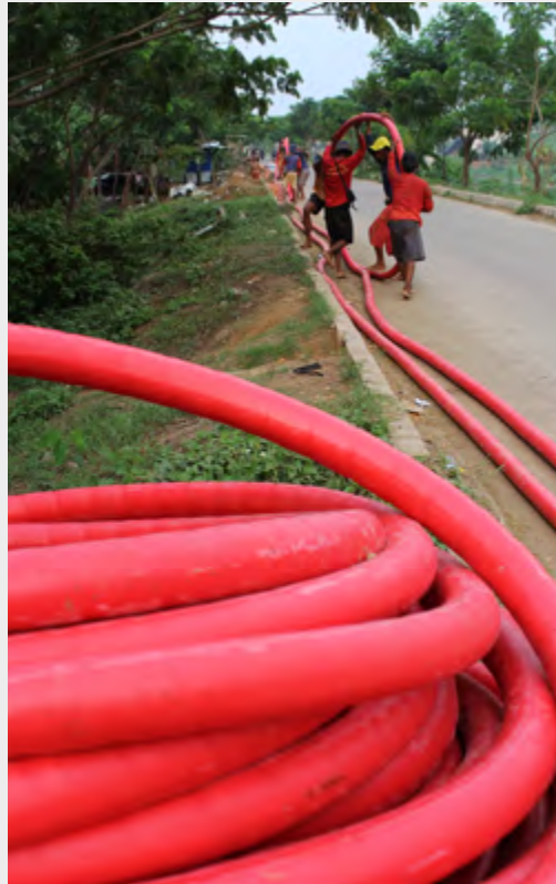
Workers laying underground electrical power lines in Jakarta Indonesia. Credit: © Yamtono_Sardi/istock.com
